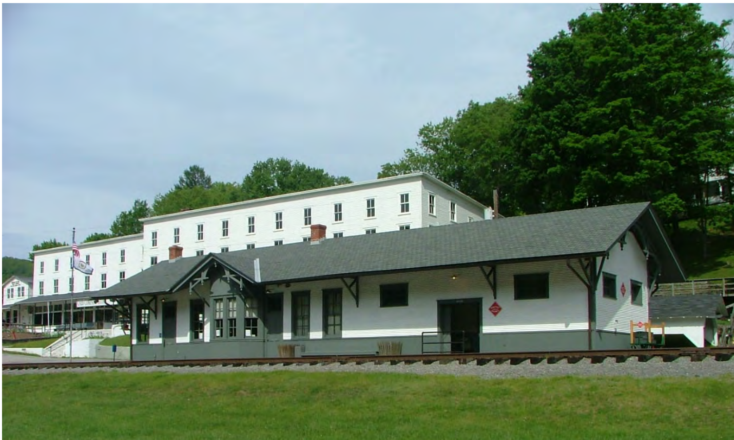
Cass Railroad Station May 2010
